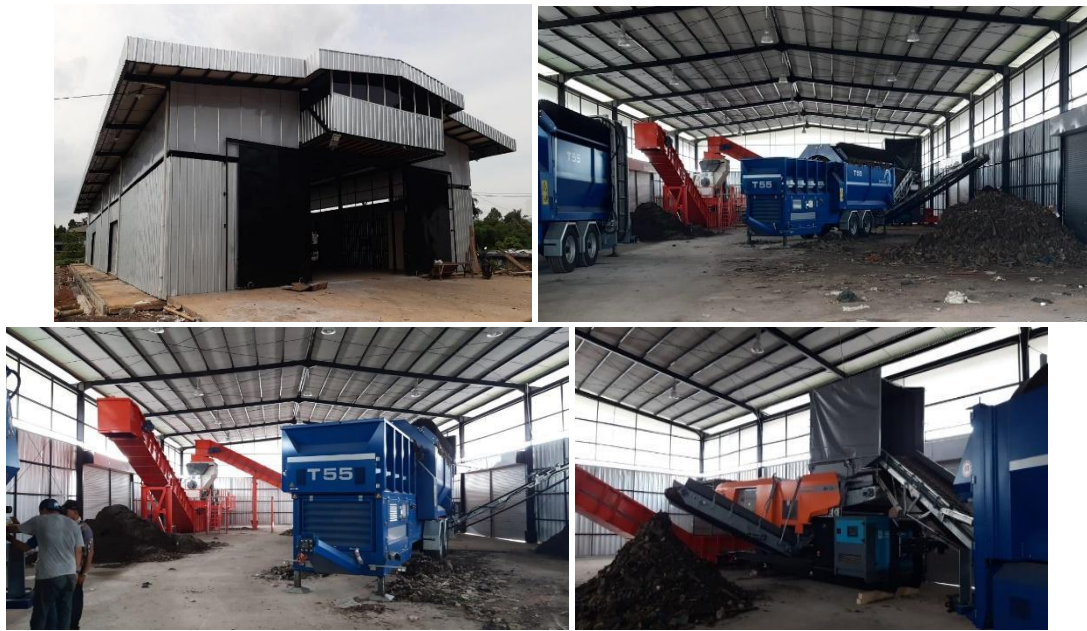
Gambar II.14. Hanggar Landfill Mining TPST Bantargebang
